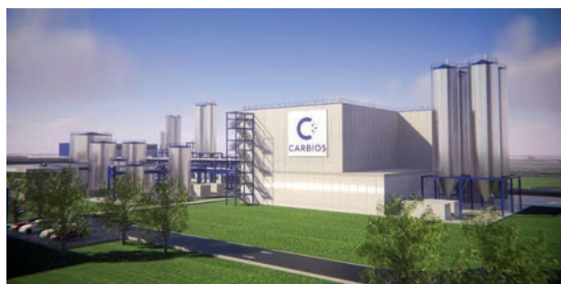
3D modeling of the Carbios industrial unit for the depolymerization of PET plastic and textile waste into monomers (credit: Technip Energies)
